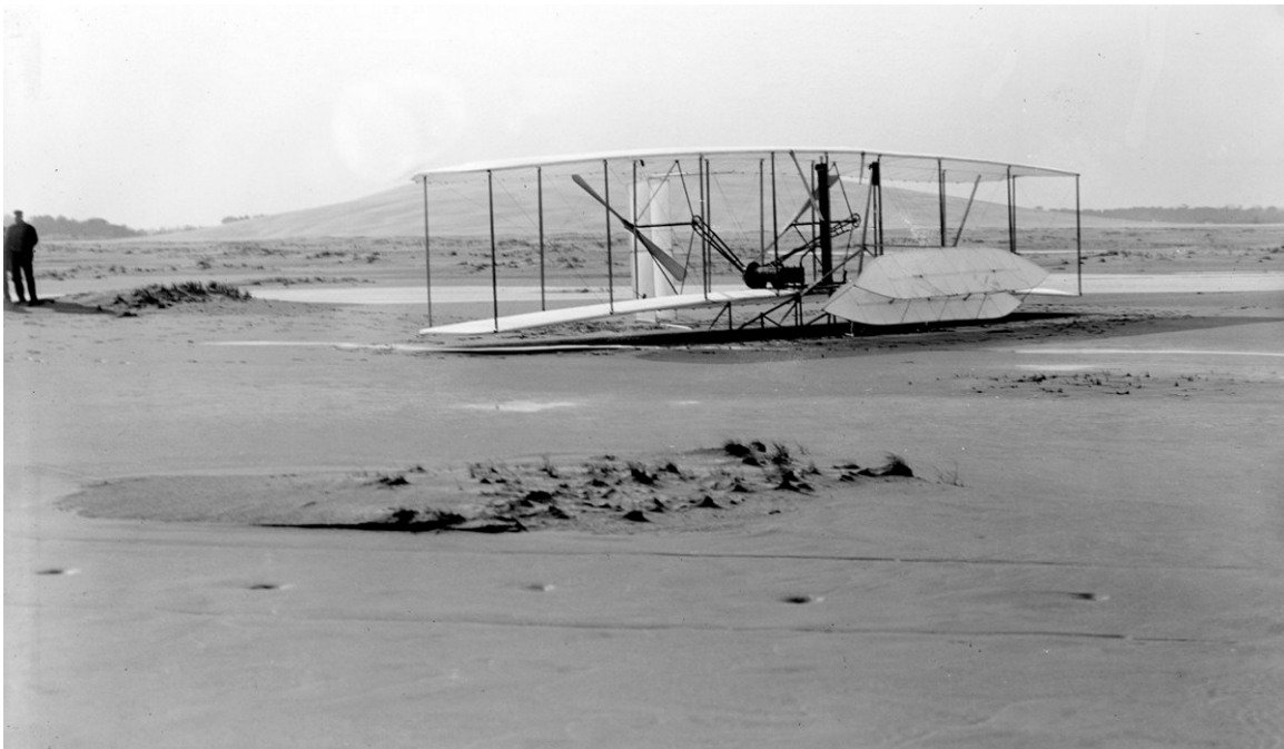
Fig. 5.9 The 4th flight of the Wright brothers at Kitty Hawk, NC on Dec. 17, 1903 ended in a crash! The forward elevators are broken. The first flight set the record. (Library of Congress LC-DIG-ppprs-00614).
